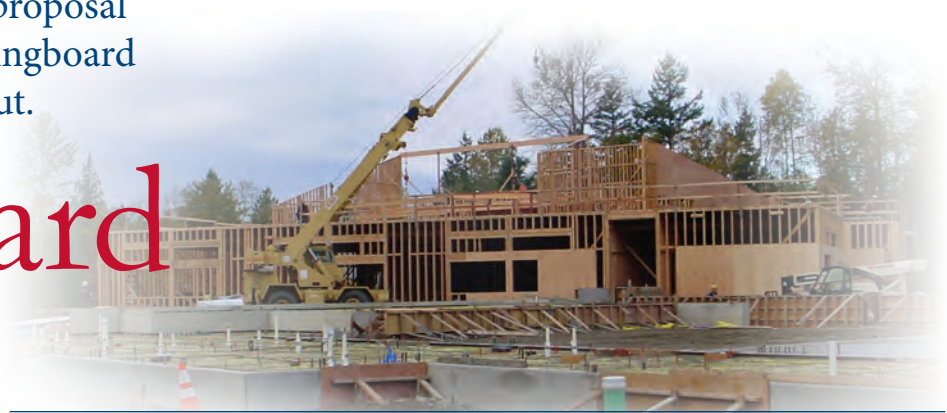
Cordata Elementary School construction will be complete this summer.
